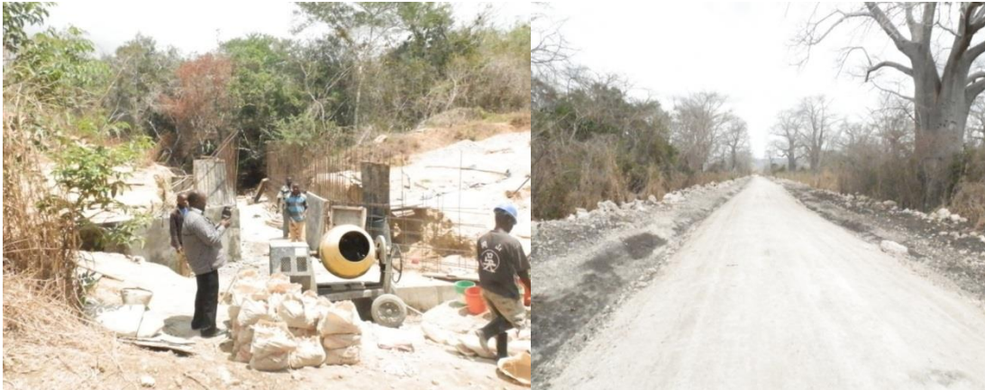
Shughuli za ujenzi, Barabara ya Mvuleni – Kitomanga
